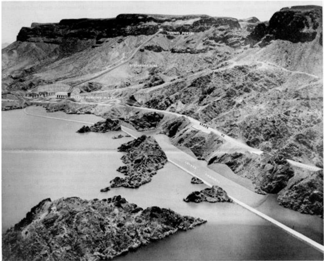
**WHERE THE DITCH BEGINS--**This artist's conception shows where water will flow into the Central Arizona Project system from the Colorado River. The pumping plant, located at Lake Havasu behind Parker Dam, will lift the water 820 feet. From there it will flow by gravity to Phoenix, thence to Pinal County and Tucson. (Bureau of Reclamation Photo.)
